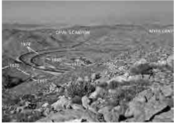
Mountain Springs Open Air Museum of Road Construction. Author's Collection.
