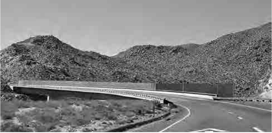
Wind Fence on Devil's Canyon Bridge No. 1. Author's collection.
