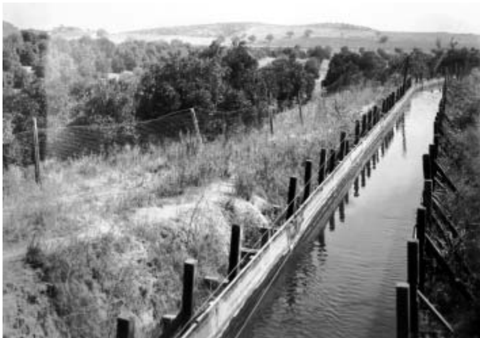
San Diego flume running adjacent to groves. Courtesy of the Helix Water District Archives.
