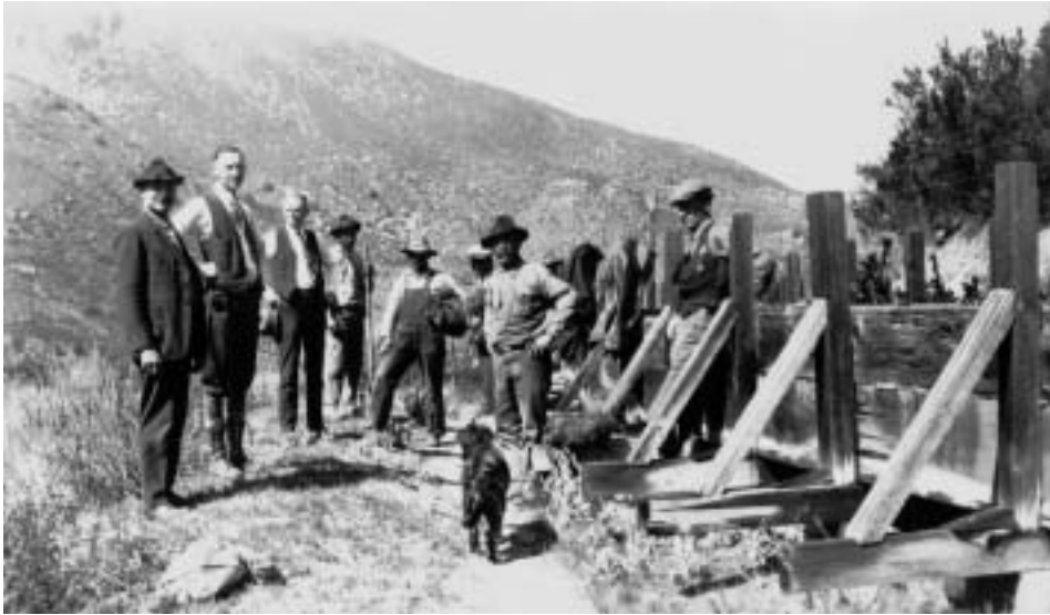
1925 flume inspection. Left to right: Chet Harritt, CWC engineer Tom King, Ed Fletcher. Courtesy of the Helix Water District Archives.
