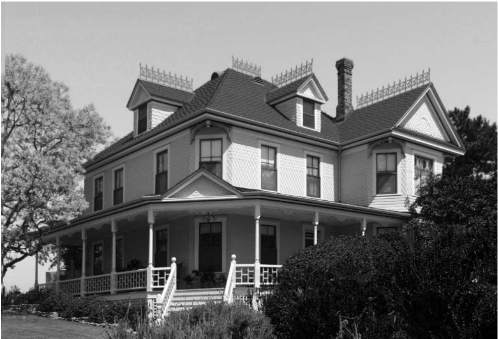
Oliver H. Noyes house restored. It is presently owned by the International Community Foundation. Photo by Steven Schoenherr.
