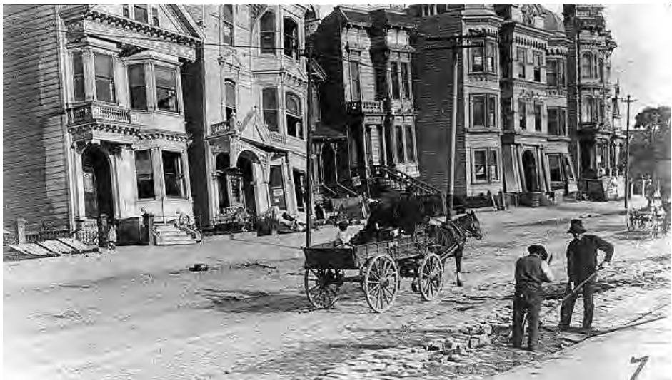
San Francisco earthquake aftermath. Photo courtesy of the Library of Congress.
