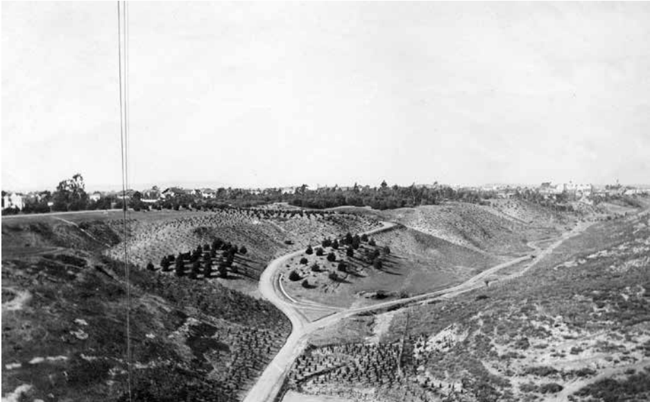
Cooke overcame the challenges of building a connecting road from Florida Canyon to the higher central mesa in Balboa Park, shown here in 1913. ©SDHC OP #16920-2.
