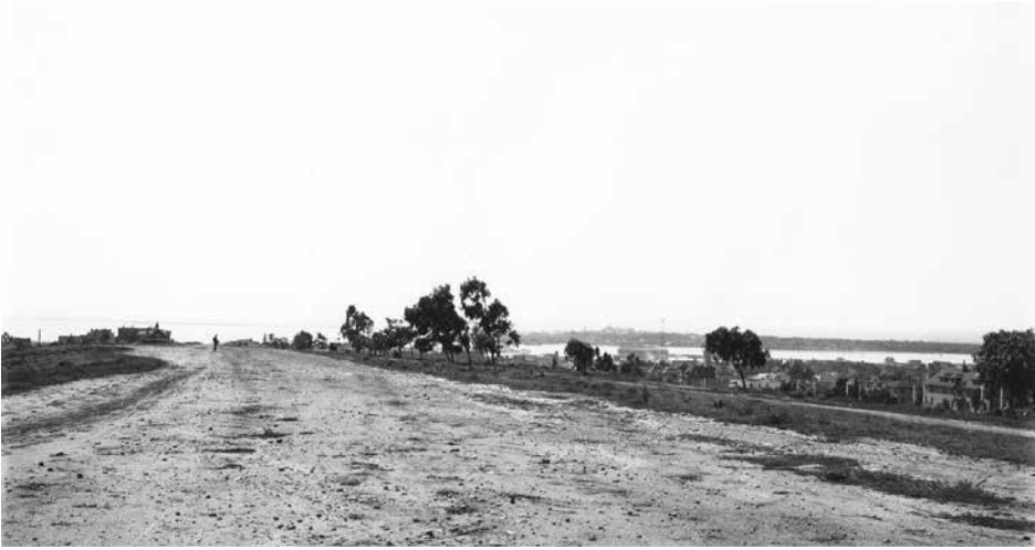
Inspiration Point road overlooking San Diego Bay under construction, 1903. ©SDHC #2434.
